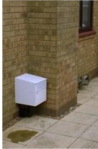
External sub-slab depressurization low level exhaust
